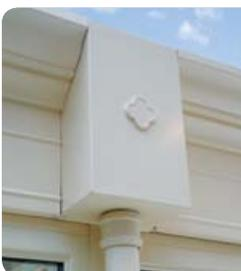
Gutter outlets are fully sealed and can accommodate a full range of decorative aluminium hoppers and downpipes.
