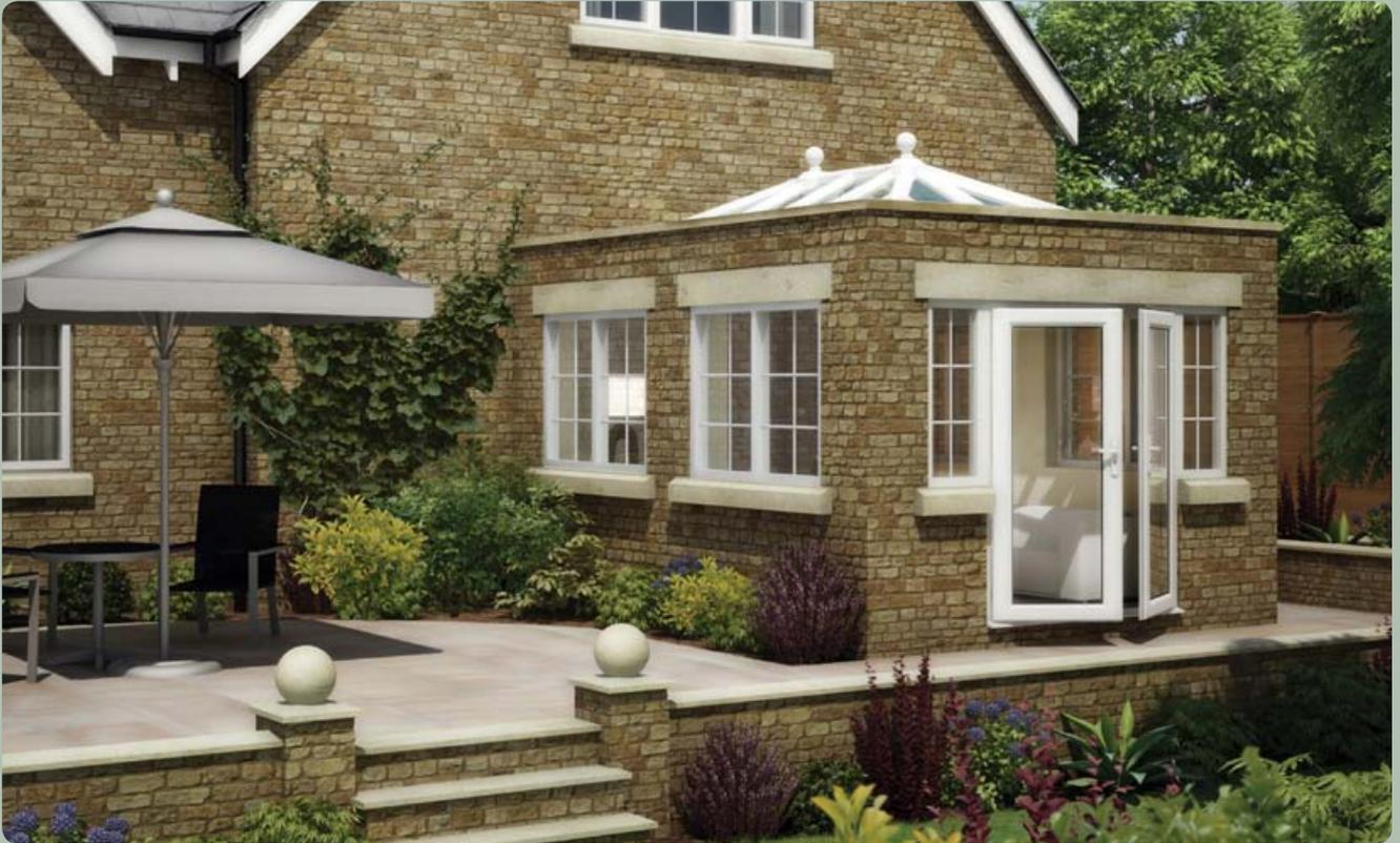
The Integra system features an insulated “warm roof” construction that fully meets all Building Regulations and utilises modern materials to best effect – high strength structural aluminium replaces timber, and an integrated aluminium gutter replaces traditional flat roof membranes. The perimeter gutter has a polyester powder coat external finish and can be walked on in safety for maintenance purposes, due to the strength of the construction.
